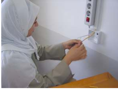
Cable installation, CS Faculty, Herat University, 2005
