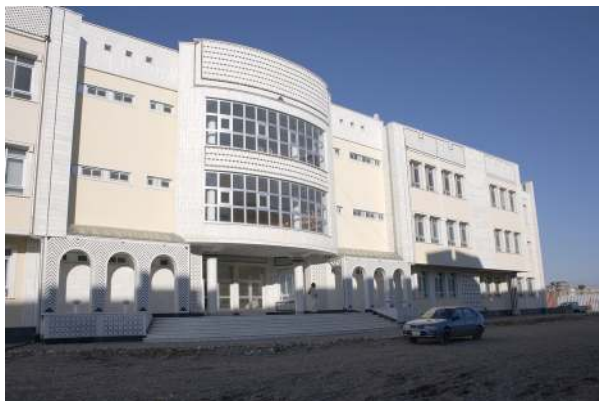
New constructon for CS Faculty, Herat University, 2021
