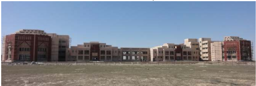
New construction, Balkh University campus, 2012
